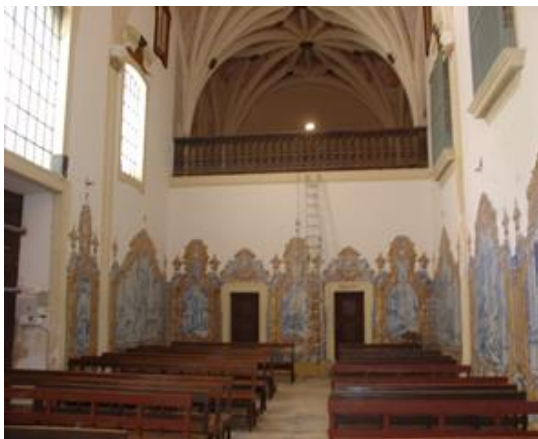
Fig. 5. Higher choir viewed from the nave.
